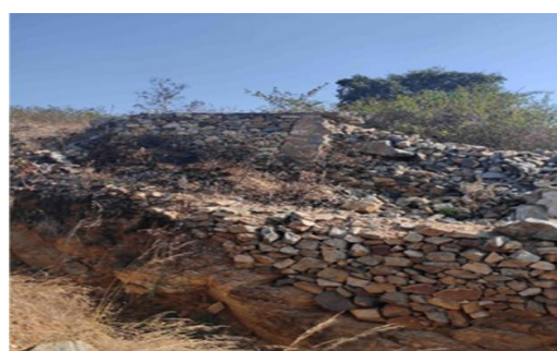
Rubble Stone Wall
