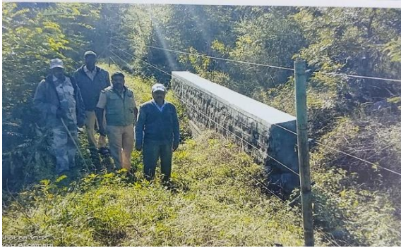
Combination of Solar fencing with RCC in K Gudi
