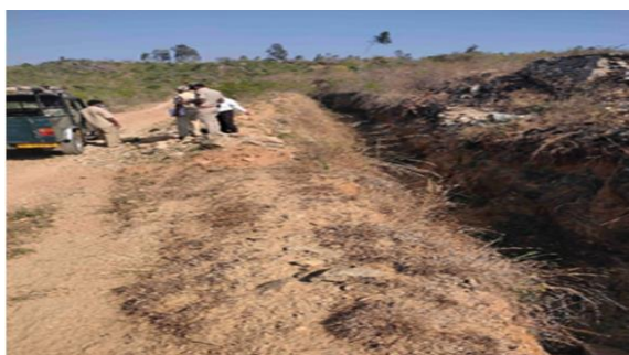
Well maintained EPT
