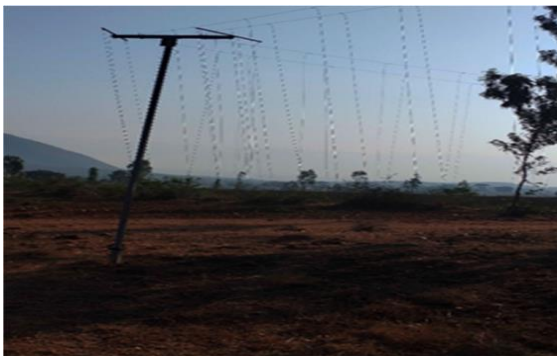
A tentacle solar fencing on the boundary of forest
