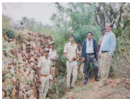
Rubble stone wall at Cowdalli range
