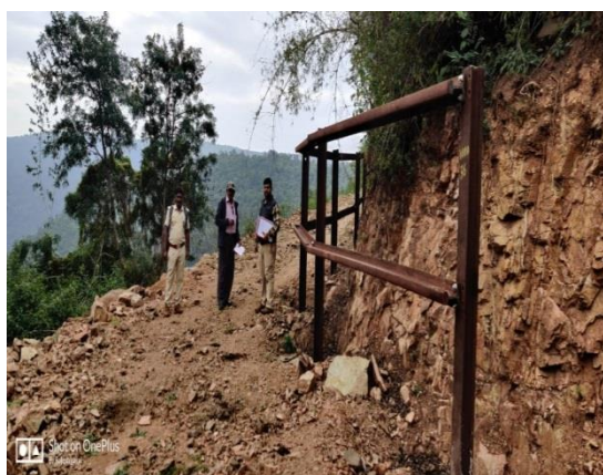
Rail fence at MM Hills Range
